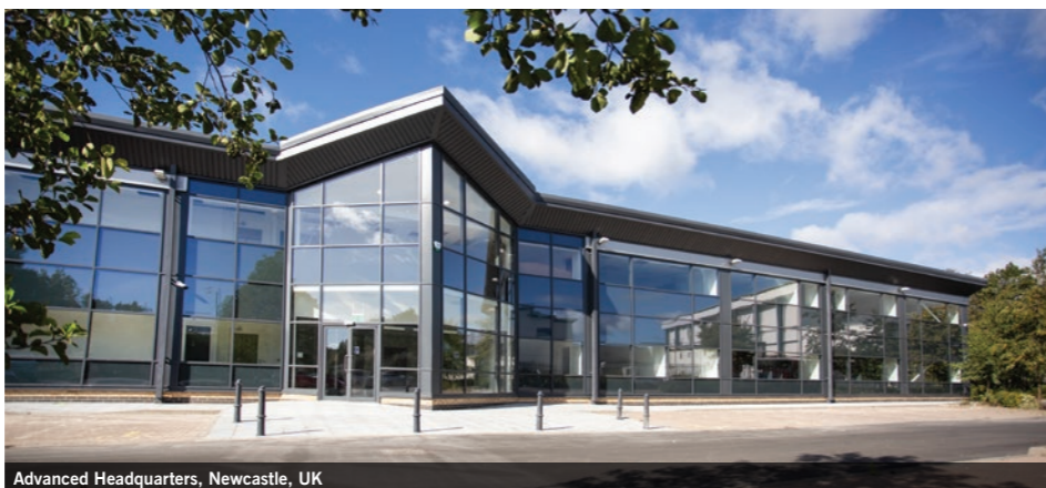
Advanced Headquarters, Newcastle, UK
