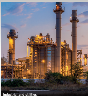
Industrial and utilities
