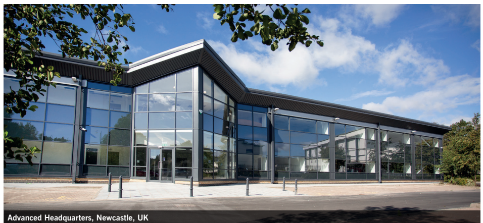
Advanced Headquarters, Newcastle, UK
