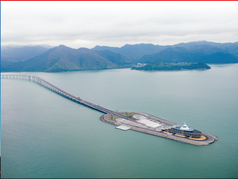
Hong Kong-Zhuhai-Macau Bridge, Hong Kong
