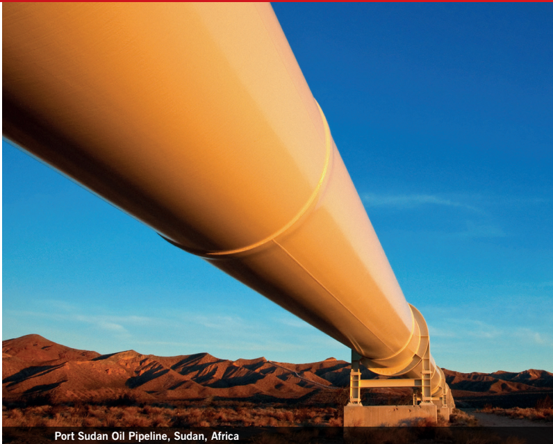
Port Sudan Oil Pipeline, Sudan, Africa
