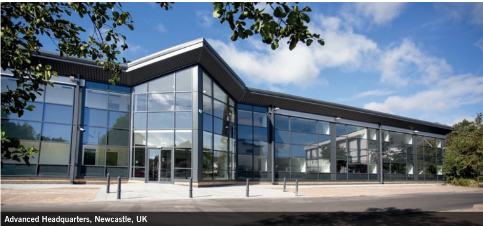
Advanced Headquarters, Newcastle, UK
