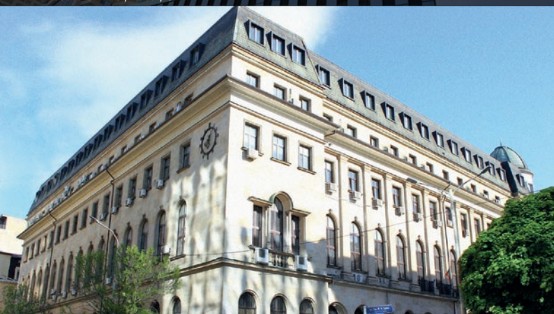
Communications Regulation Commission office, Sofia, Bulgaria
