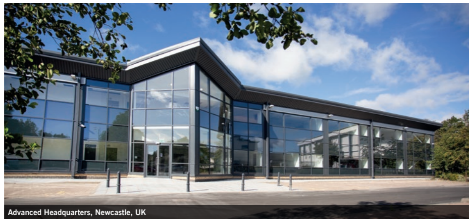
Advanced Headquarters, Newcastle, UK
